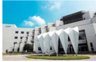
Tainan Plant (Diamond-rated Green Building)
